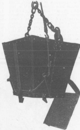
Bucket With Rope Tripping Device (Open)
