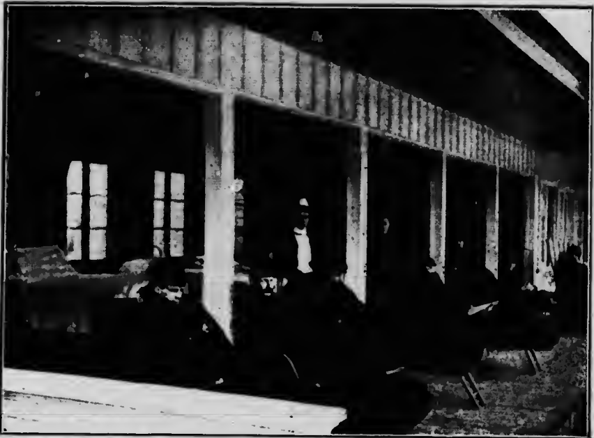
THE MOUNTAIN SANATORIUM: MEN'S SHACK.
