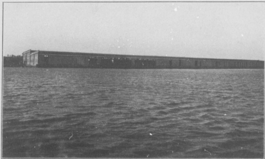
C.P.R. Warehouse, 1,150 feet long. There is another completed 750 feet long.
