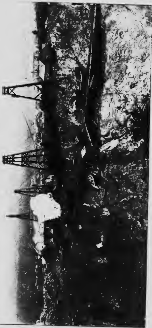
Arrangement of Cable Derricks and Tracks near Border of Pit, King Bros. Mine, Thetford.
