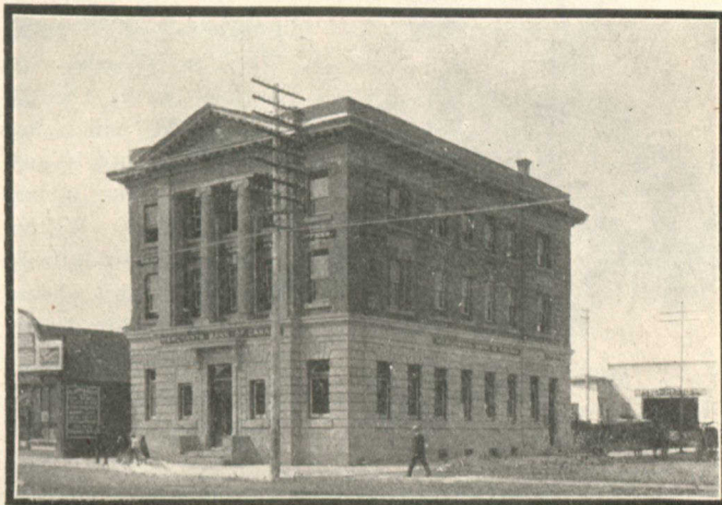
Merchants Bank. (Divisional Offices of G.T.P. on third floor)
