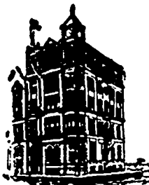
HEAD OFFICE BUILDING, MONTREAL.
