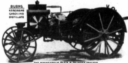
THE MINNEAPOLIS 15 H.P. 4-CYLINDER TRACTOR ALL GEAR ENCLOSED AND RUN IN OIL
