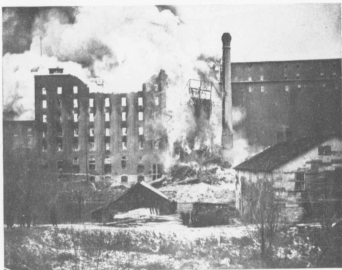
Fig. 4. Shows collapse of grain tank and dry house; also fire gaining headway in frame metal clad grain elevator.
