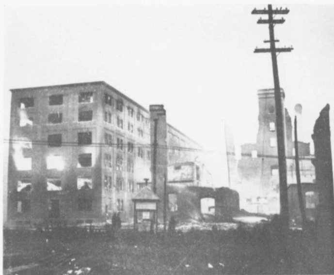
Fig. 8. View looking North from Hunter Street. Note stock piled high in concrete warehouse. Ruins of mill buildings on right.
