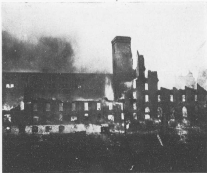
Fig. 7. Shows how concrete warehouse, equipped with wired glass windows, withstood exposure until other buildings collapsed.
