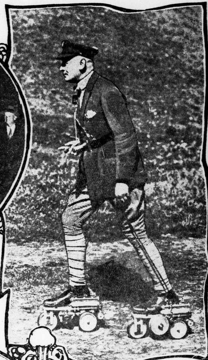
SOMETHING NEW — Gebhardt, noted automotive engineer of Munich, Germany, demonstrating his power roller skates, which are propelled by tiny acetylene-gasoline motors. He is at present at work on a new type of improved aeroplane engine.
