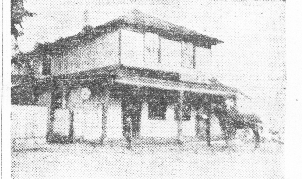
Graham Hotel, on Hamilton road, near which Fred Culver was killed following a fight in the barroom. The Whitney license commissioners received following a fight in the barroom. The Whitney license commissioners received following a fight in the barroom. The Whitney license commissioners received following a fight in the barroom.
