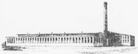
The Dominion Linen Mills (under construction), Bracebridge.
