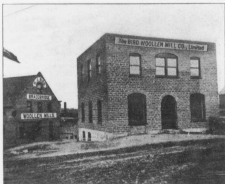
The Bird Woollen Mill, Bracebridge.
