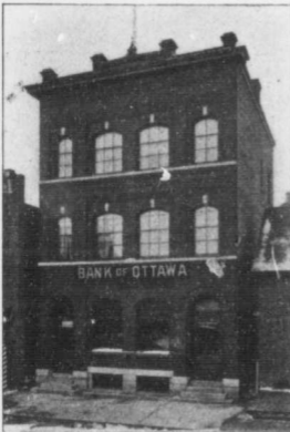
Bank of Ottawa, Bracebridge.
