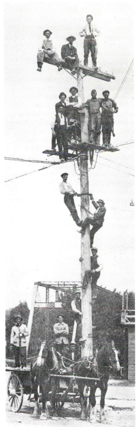
Telephone linemen became the heroes to small boys and bustle-clad women at the turn of the century and sometimes they liked to show off, as shown in the above photograph, by climbing up a telephone pole. They used horses and wagon to carry equipment and often walked miles for repairs and for stringing new lines across the country.
