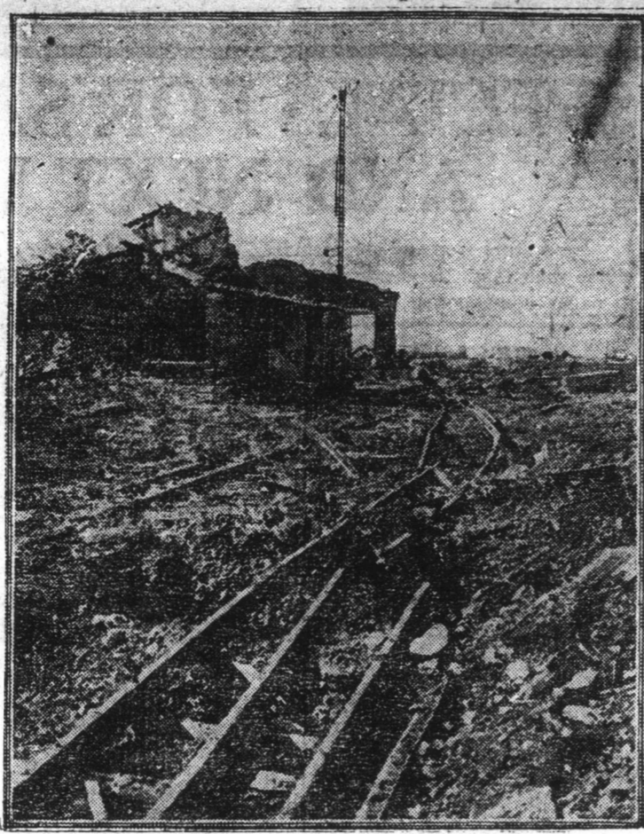
RAILWAYS DISAPPEAR UNDER LONG BOMBARDMENT. The task of bridging the crater area is one of the most important which confronts our armies in the west. Here is an example of a station with its adjacent railway lines and sidings in a state of partial obliteration. It is the only task of the army railway builders to replace these lost lines as rapidly as possible.
