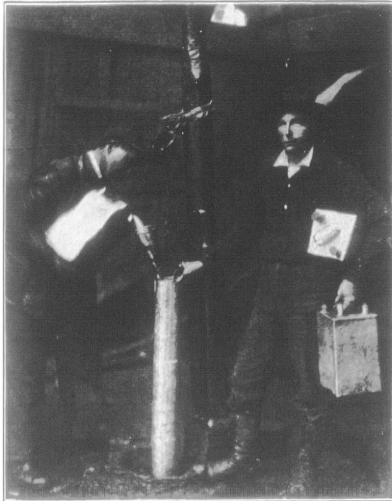
Pouring Nitro-glycerine into the cylinders to lower into Well for "Shooting" the Oil Sands.
