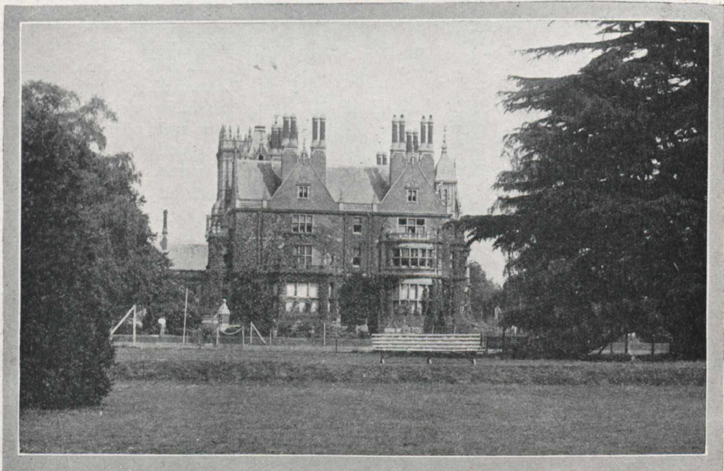
View Across West Terrace.
