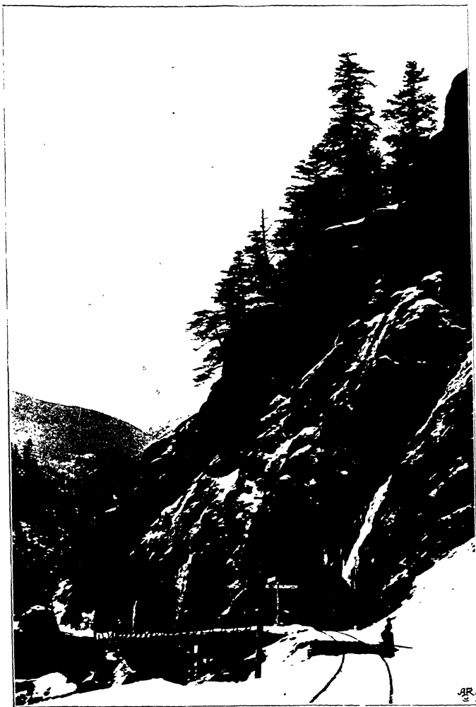
WAGON ROAD AROUND BLUFF—RAILWAY TUNNEL THROUGH IT.
