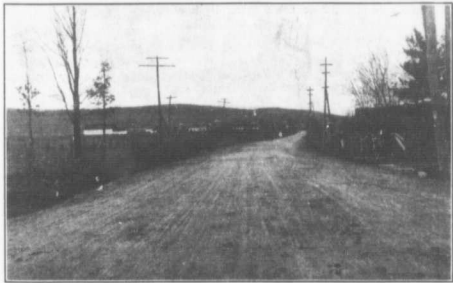
Roads, Such as This One, are Appreciated at This Season
