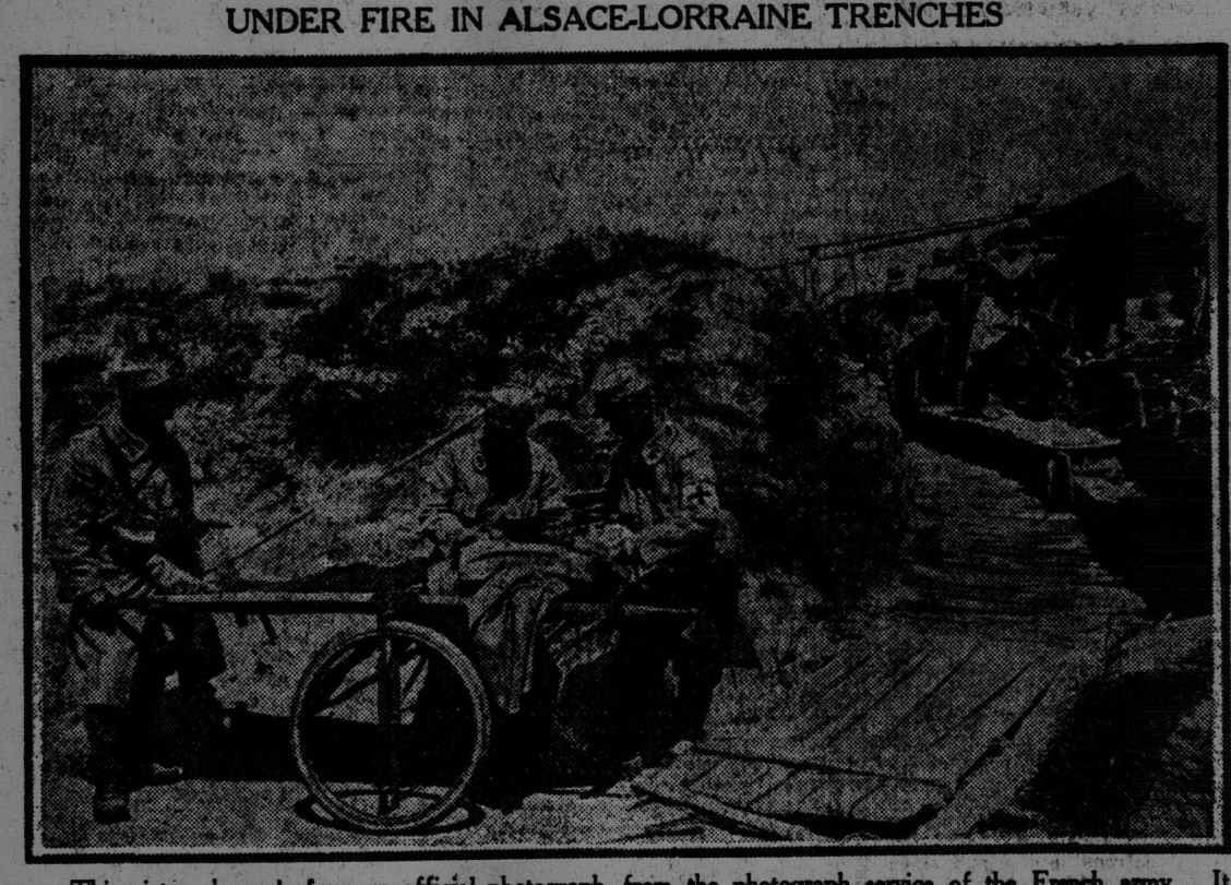
UNDER FIRE IN ALSACE-LORRAINE TRENCHES. This picture is made from an official photograph from the photograph service of the French army. It was taken in actual battle and shows Red Cross men removing a wounded soldier while his comrades, at loopholes, are firing on the enemy.
