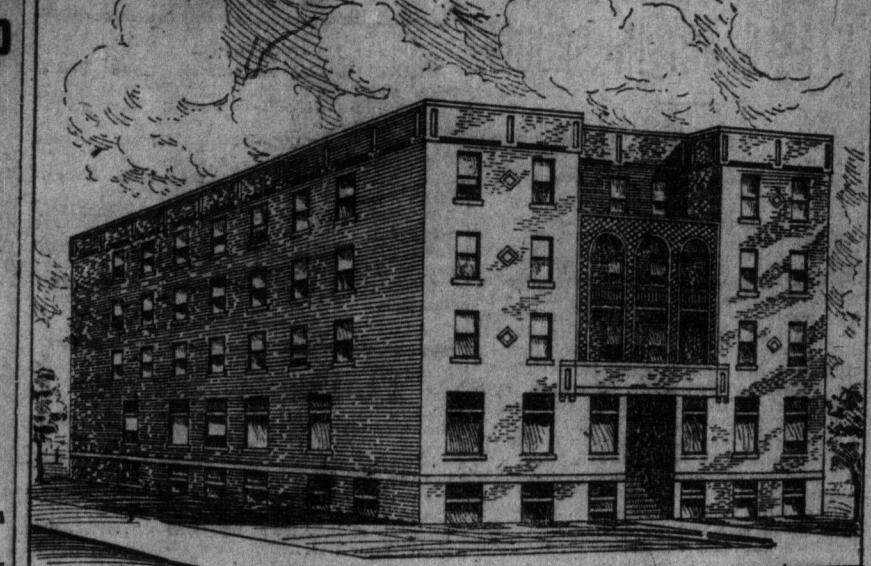
NEW Y. W. C. A. BUILDING UNDER CONSTRUCTION AT THE CORNER OF ST. PATRICK AND CASIMIR STREETS. EARL GREY WILL OFFICIATE AT ITS DEDICATION THIS MORNING.
