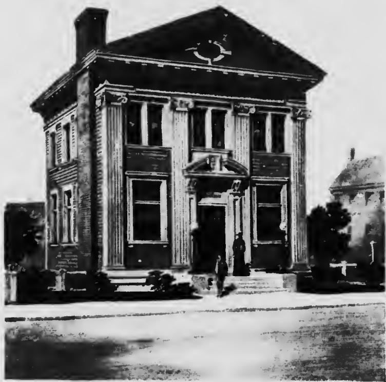
CARMAN, MAN. Under construction
