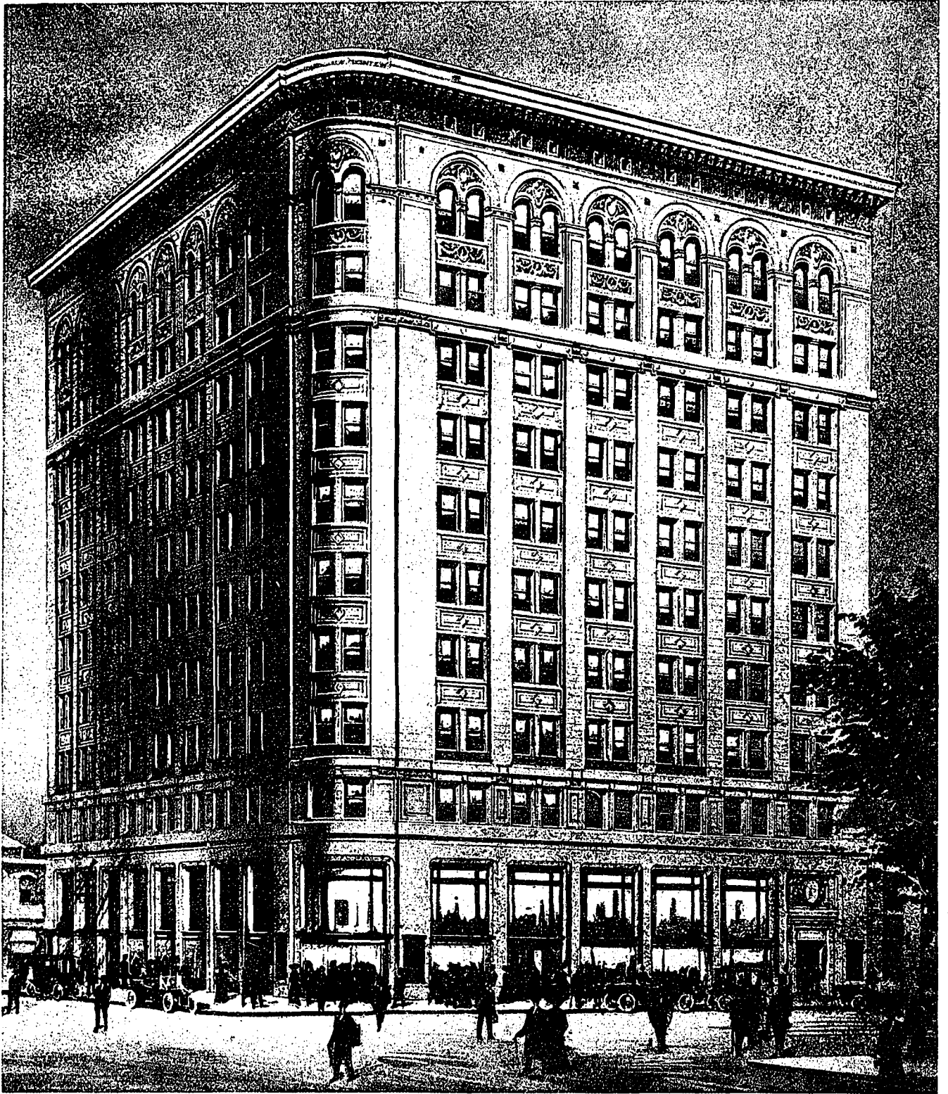
BIRKS BUILDING, VANCOUVER, B.C.
