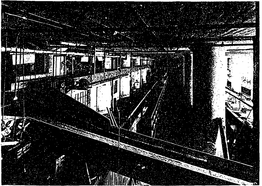
MEZZANINE VIEW SHOWING CONVEYOR AND PARCEL CHUTE.
