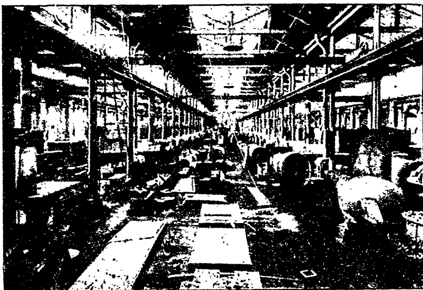
BOILER SHOP, CREWE WORKS.
