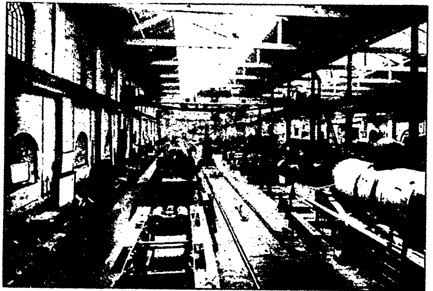
ERECTING SHOP, CREWE WORKS.
