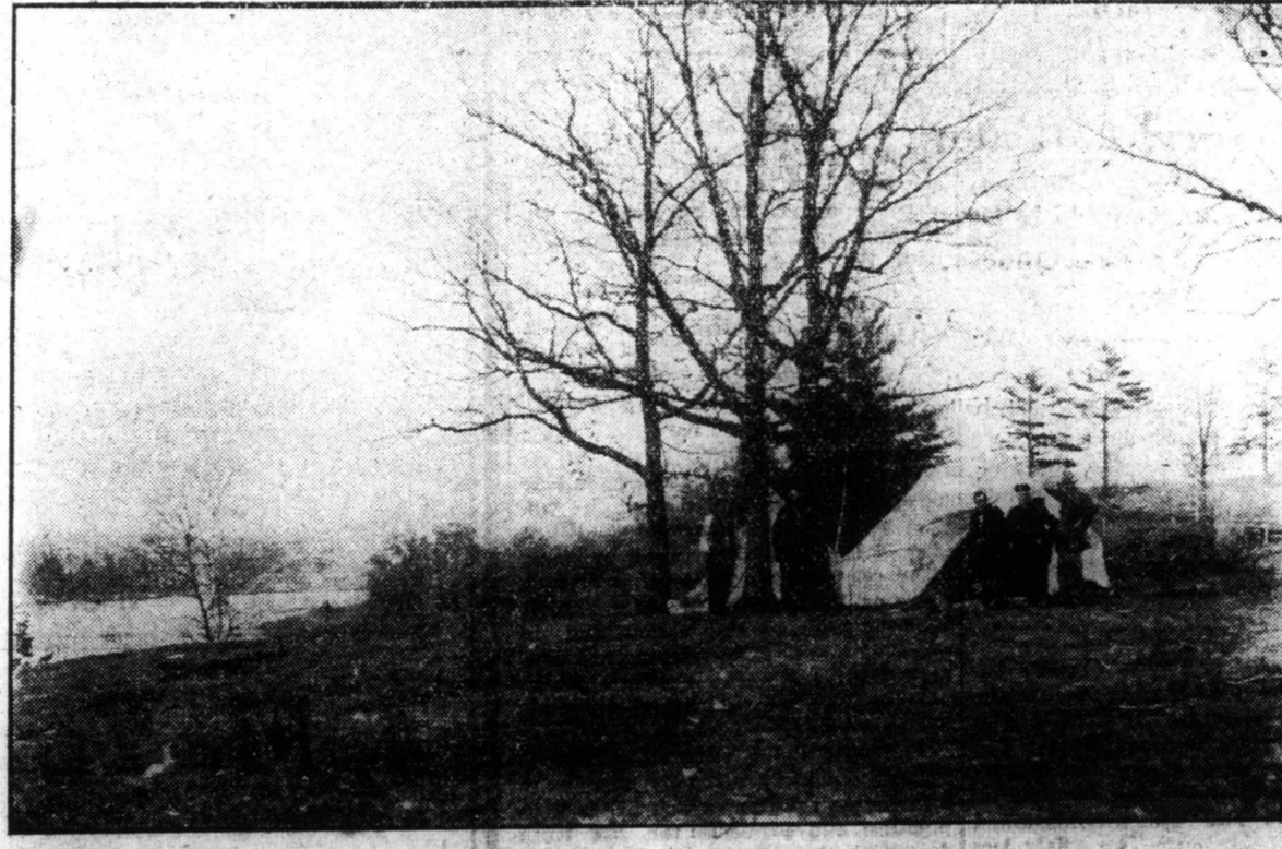
Scene near Paris of a portion of the construction camp and another beautiful adjacent view of the river.
