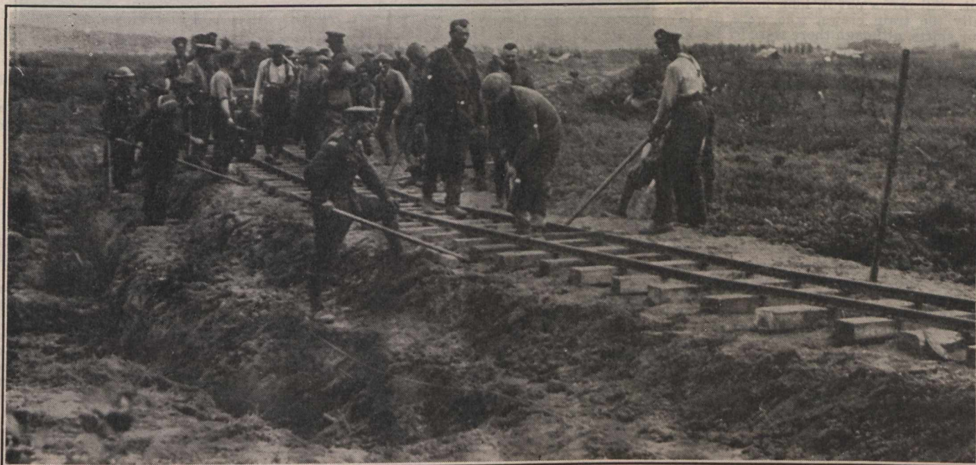
Track Gang on Light Railway Construction.
