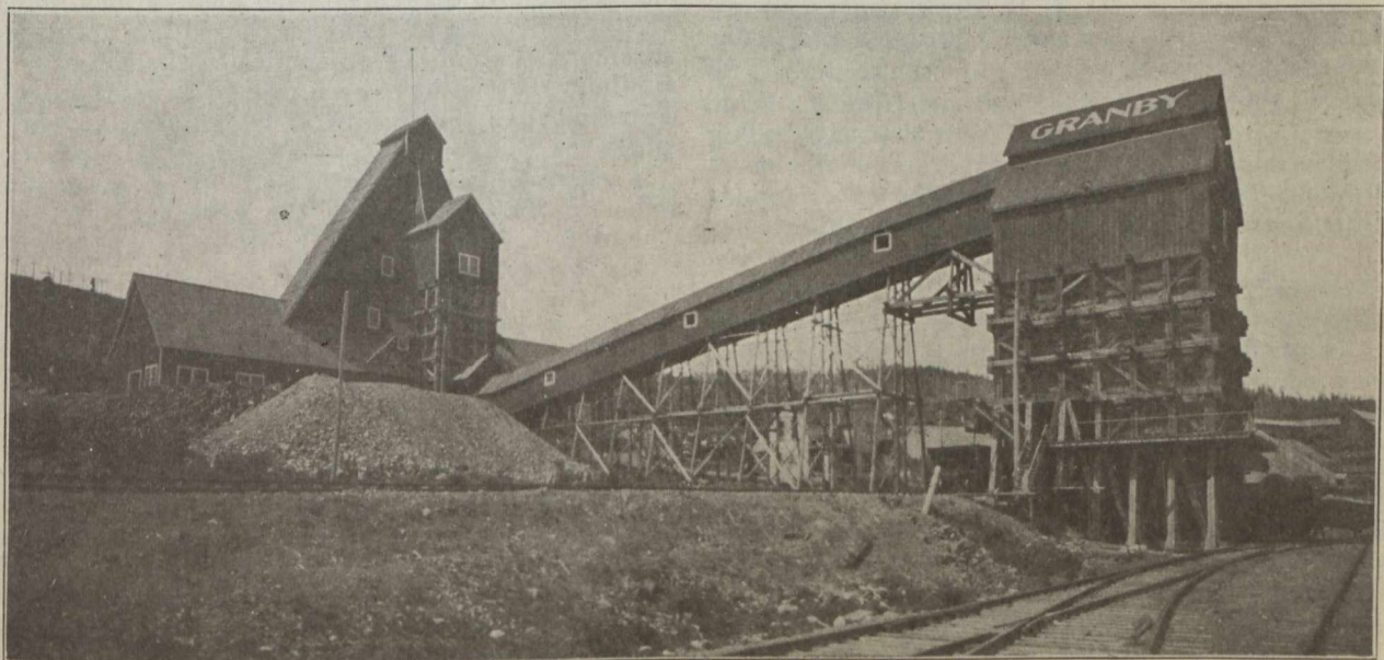
Victoria shaft terminals on C.P. and G.N. Railways—Granby Consolidated, Phoenix, B.C. Over 10,000,000 tons of ore have been shipped from the Granby Mines at Phoenix.
