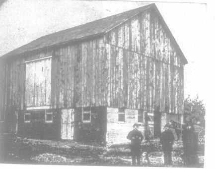
Size, 36x46 feet. Basement built with Thorold Cement.
