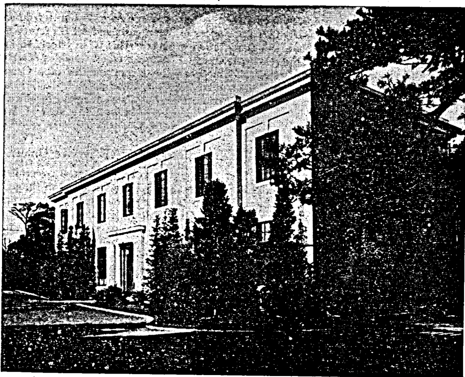
The chancery building, Canadian embassy, Tokyo, Japan.
