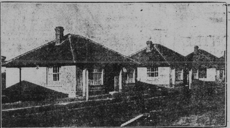
Here are some of the houses erected by the British Red-Cross Society at Norwich for disabled soldiers. They contain every labor-saving device known to modern science.
