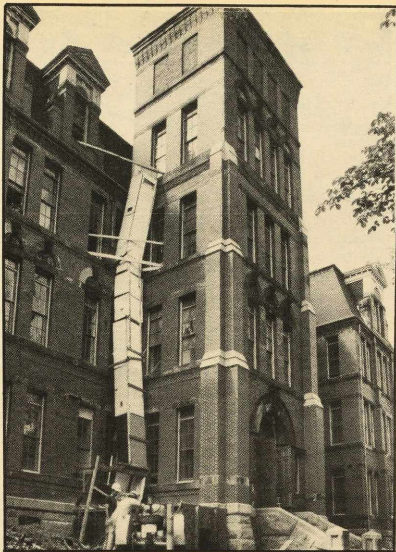
Forrest building under reconstruction in 1983. Photo by Carlos, Dal News.
