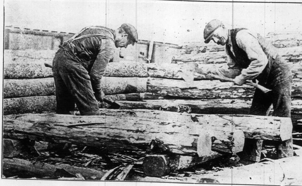
STRIPPING BARK OFF TIES IN THE AGINCOURT YARDS FOR THE C. P.'S LAKE FRONTLINE.
