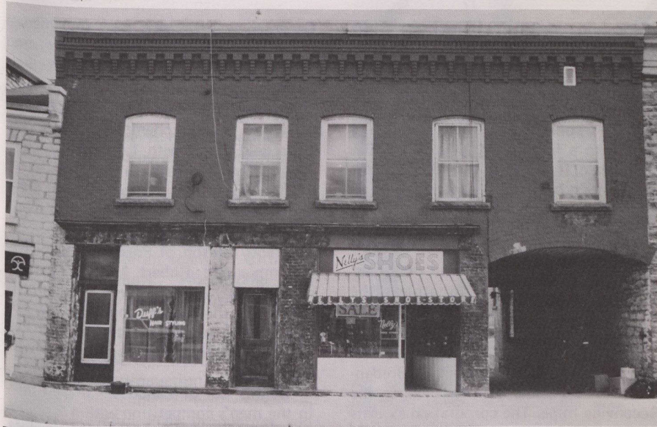
Two shops on the main street in Perth before renovation.
