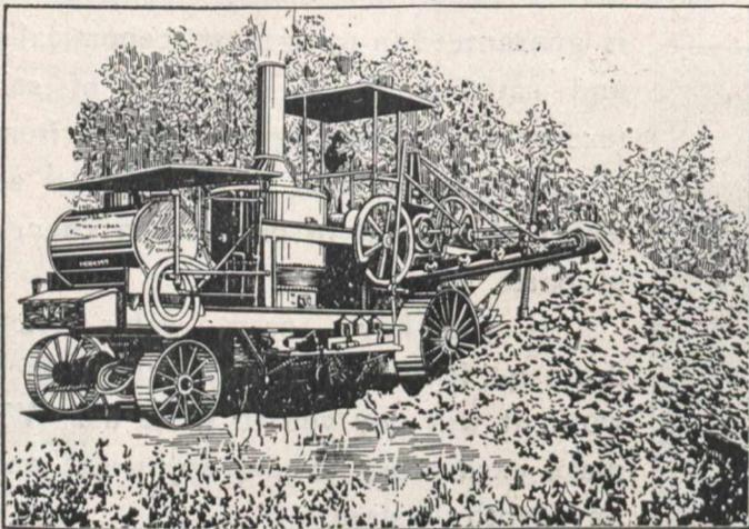
Trench Excavation is about the most severe and exacting work to which a Machine Excavator can be put.
