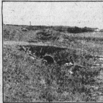
Method of Carrying Terrace Water Under a Roadway by Means of a Culvert.
