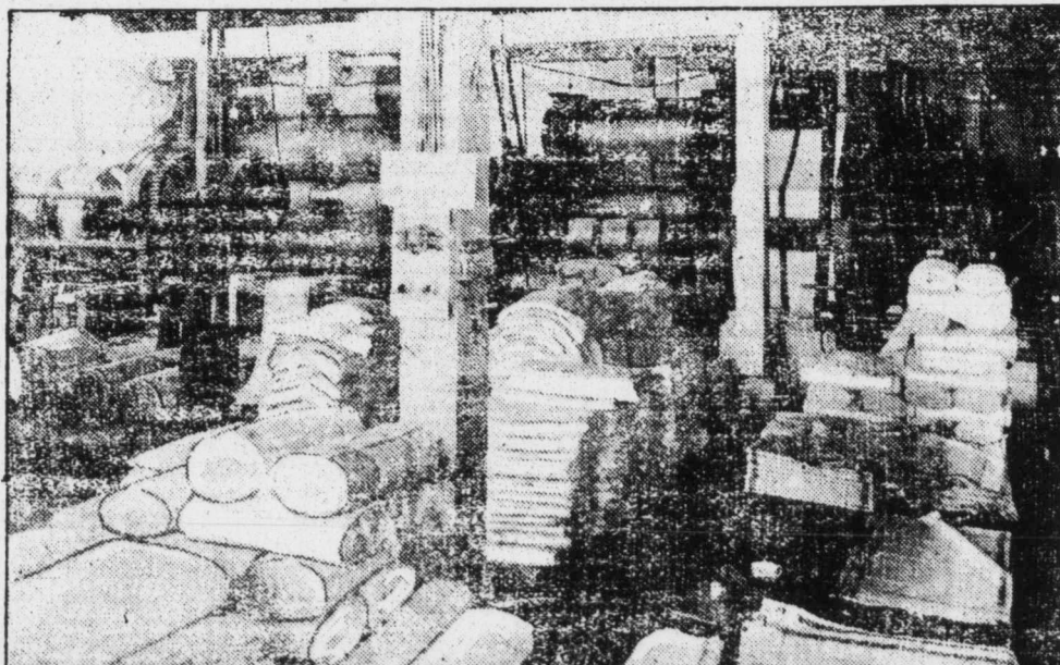
Dominion Linens, Ltd., Mangling and Ironing Department, showing Callanders, Hydraulic Mangles, Folding and Measuring Machines. Total floor space about half acre.
