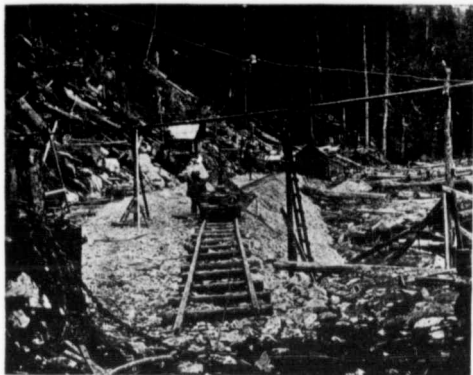
Showing Dump at Coquitlam.
