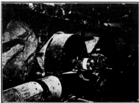
Ventilating station at Coquitlam Heading.
