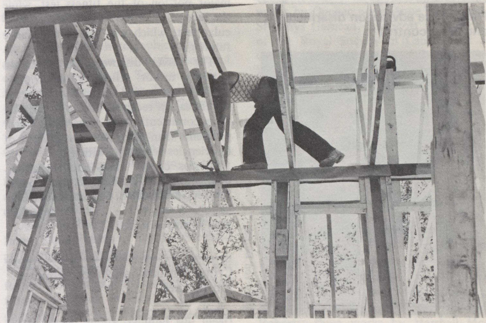
Prefabricated wood structural components are erected on site.
