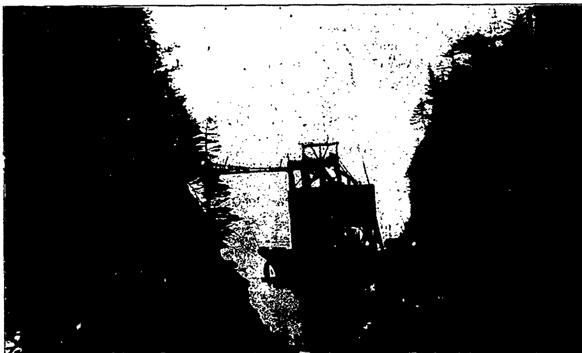
Shipping Pier, Bell Island Iron Mine, Newfoundland.
