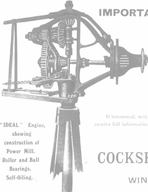
"IDEAL" Engine, showing construction of Power Mill. Roller and Ball Bearings. Self-oiling.
