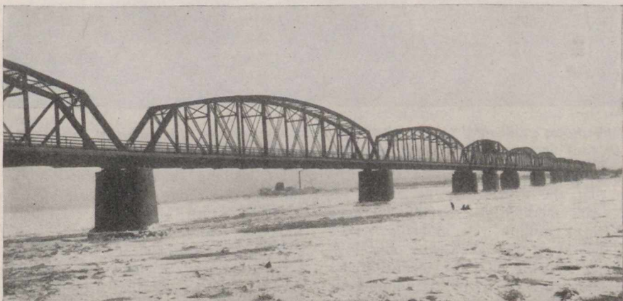
Fig. 13 represents the railway bridge over the Yalu River between Manchuria and Korea—evidently a pin-connected structure and, therefore, not quite up to the latest American practice April, 1930.
