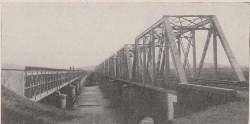
Fig. 12 shows two parallel bridges over the Toh Shi Ho on the S. Manchuria Ry. To the left, an old Russian structure; right, a modern Japanese bridge built on American principles
