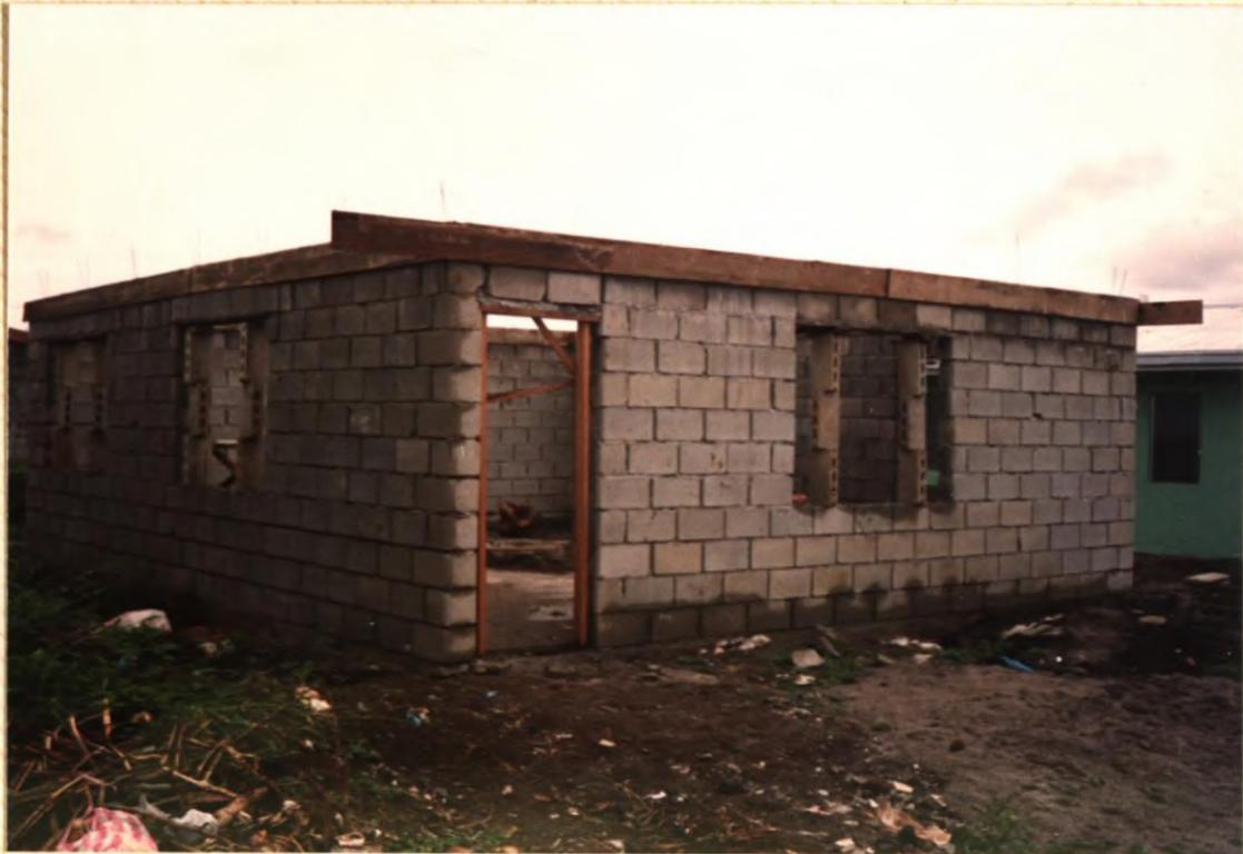
No. 61. This series of photographs, Nos. 61 to 69 will show the steps in the construction of a typical hollow-block house.
