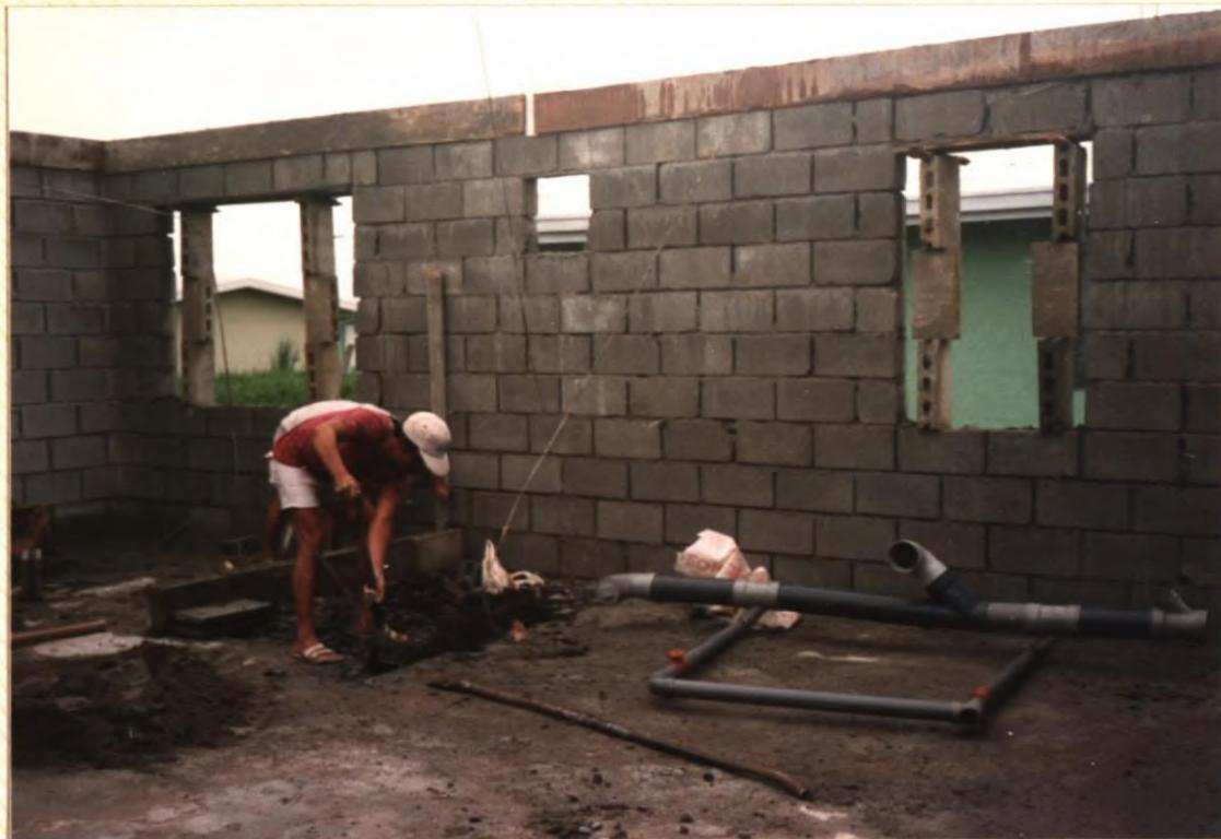
No. 62. Installing toilet plumbing. Note window header supports while concrete is curing.
