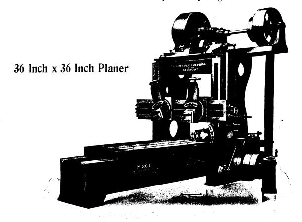
The illustration shows our 36 Inch x 36 Inch Planer arranged with three cutting heads and motor drive for Locomotive & Machine Company's Shops at Montreal.
