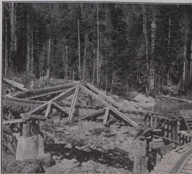
Junction of "Y" Creek Flume With Main Flume.
