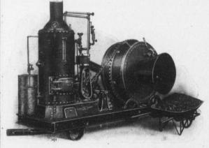
Combined with Gasoline, Steam or Electric Power. Batch Mixers, Continuous and Hand Power Mixers.
