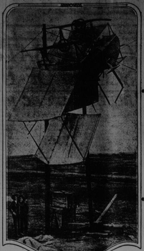
This picture, forwarded from Belgium, shows the disastrous end to a night flight by a British aviator. The poles were part of an elaborate lighting system for illuminating the field so that the pilot could make a safe landing, but the sudden blaze of light confused the pilot, with the result shown. The pilot escaped serious injury.
