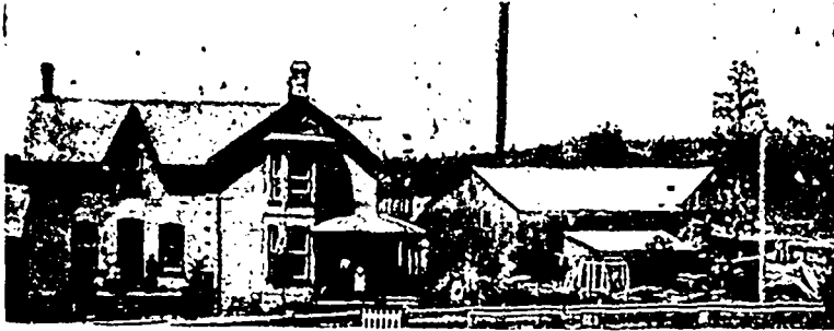
RESIDENCE AND SAW MILL OF MR. J. W. CRAWFORD, DURHAM, ONT.
