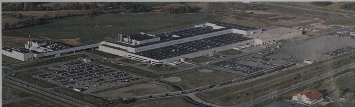
Toyota's plant in Cambridge, Ontario
