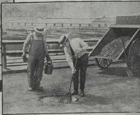
The hole to be patched is cleaned out and the bottom and sides are painted with "Tarvia-KP."
