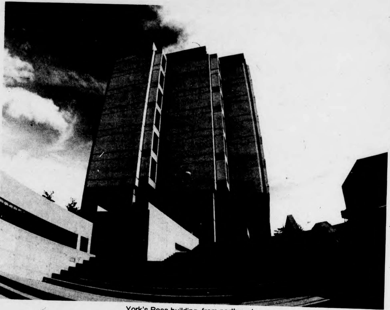
York's Ross building, from north end.
