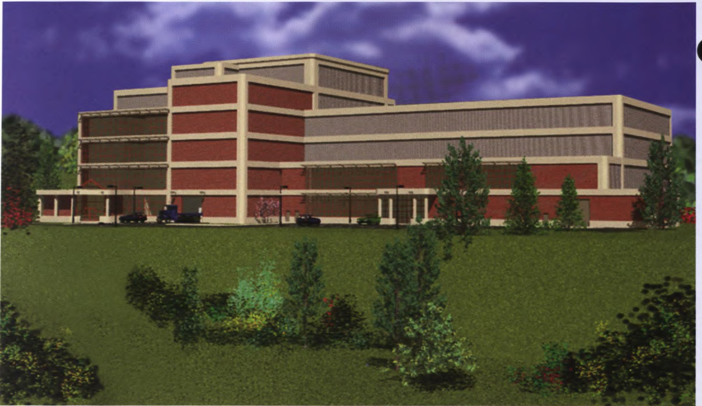
Figure 2. Artist's impression of the CNF Building, including the neutron beam guide hall on the right.
