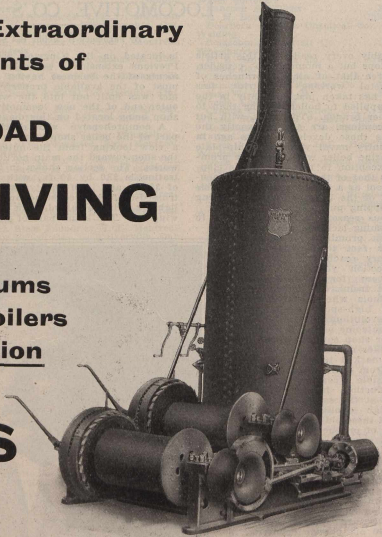
Double Cylinder Double Drum “American” Pile Driver Engine
